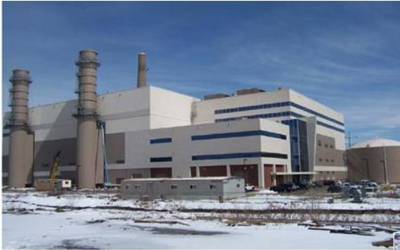
High-Bridge Combined Cycle Project, South-West Elevation – March 2008
